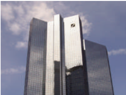
Deutsche Bank Twin Towers in Frankfurt
