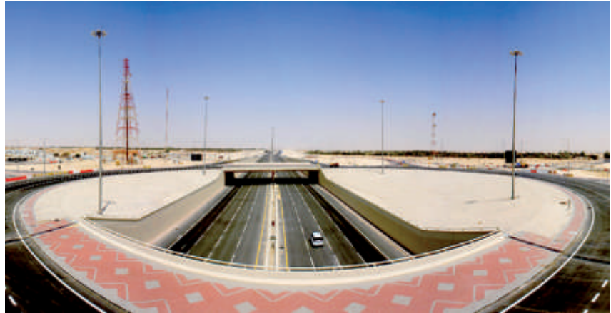
Construction site of Qatar's Expressway Programme
