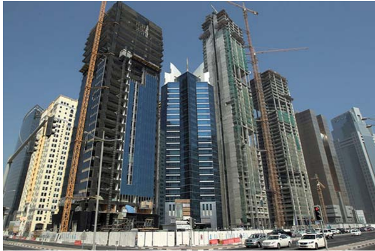
Downtown: "new office buildings and hotels under construction in the new City Centre district"
